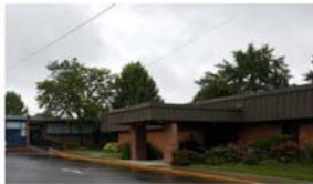
MBE Construct canopy from school to kindergarten
