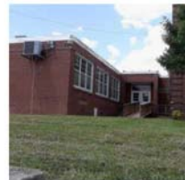
SMS Replace handicap ramp at front
