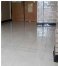
SMS Replace floor tile
