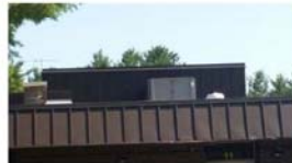
CPS HVAC Unit replacements
