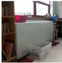
BEL Replace through-wall heating units
