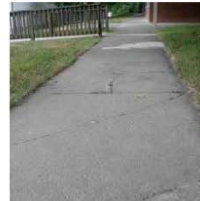
CES Replace deteriorated sidewalks
