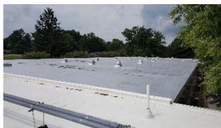
Roof Replacement Project Gilbert Linkous Elementary roof area #1
