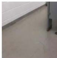
AES Replace Epoxy bathroom floors
