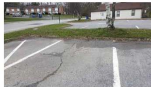
HAE Overlay/re-pave asphalt parking lots and drives, rebuild curbs, Increase number of marked and paved parking spots. Replace sidewalks
