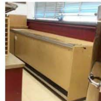
SMS Replace through-wall heating units
