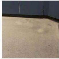
EMHS Replace Main office flooring
