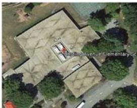
HAE HVAC Units Replacement
