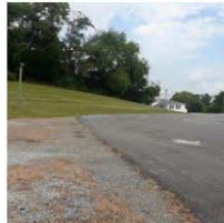
CES Additional Asphalt for parking
